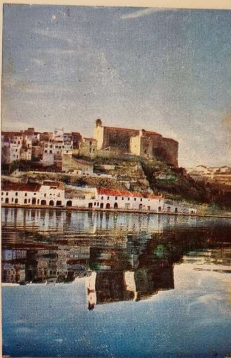
Mahón. Detalle del puerto. Al fondo la iglesia y ex-convento de San Francisco. Detail of the port. In the background the church and former Friary of St. Francis.
